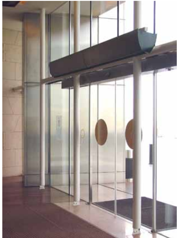
Two units can be installed together with a joining kit to form a continuous air curtain above a wide doorway.
